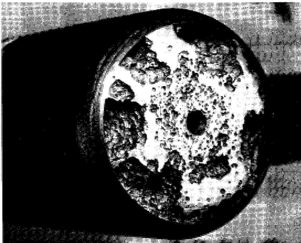
Figure 1.1-5. Selective galvanic corrosion of aluminum encased in steel.
